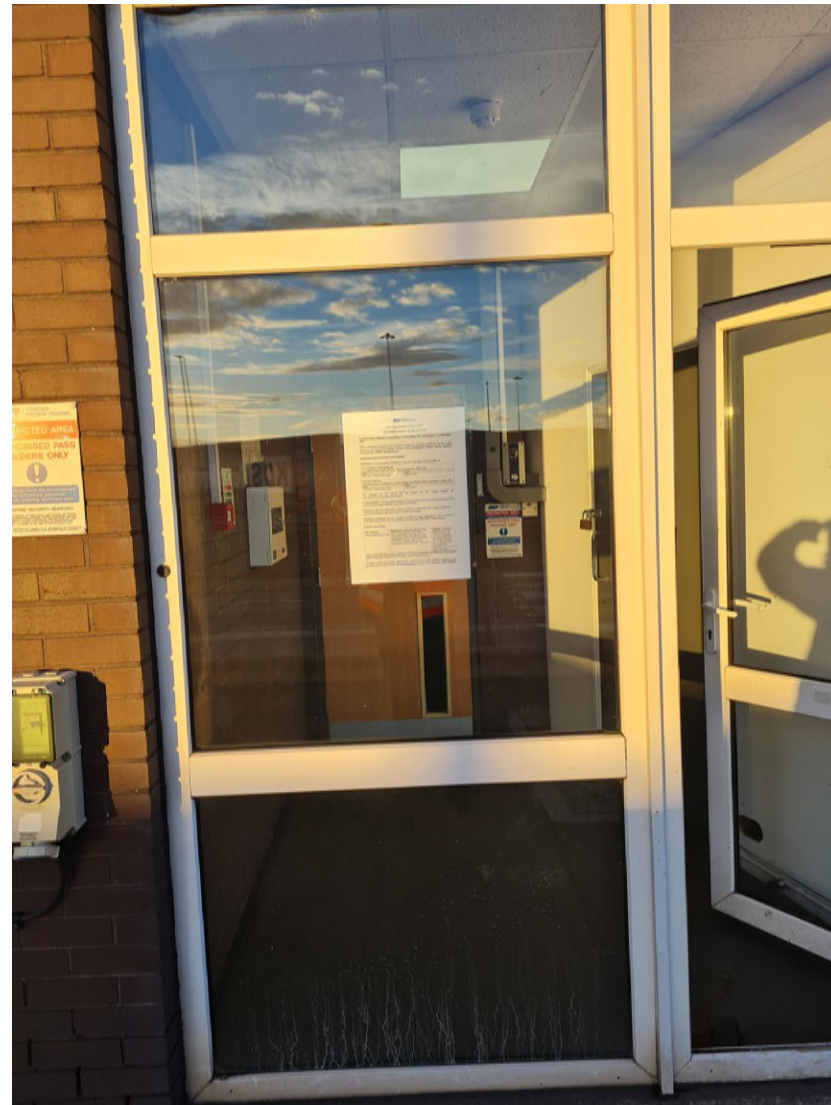
Immingham Container Terminal – Main Visitor Reception (Close up)
