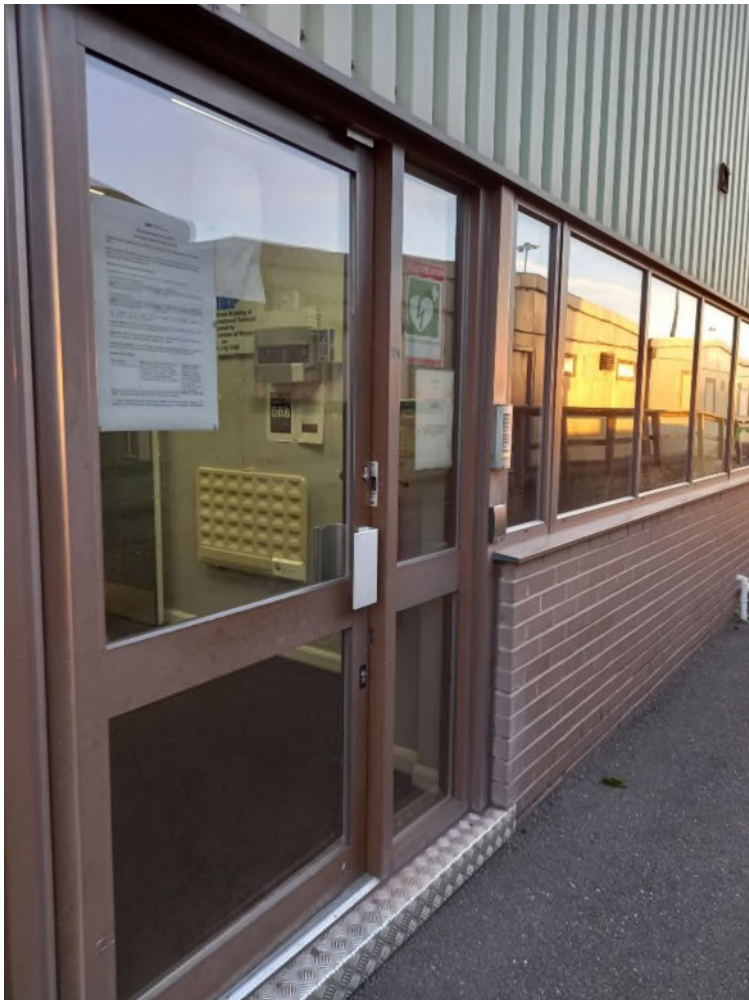
Humber International Terminal – Main Entrance to offices
